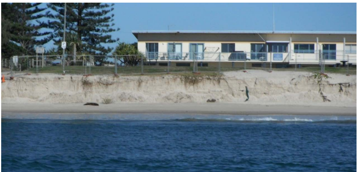
Plate 6: Recent beach erosion in front of the Evans Head SLSC (Photo by G. Owers, August 2012)
