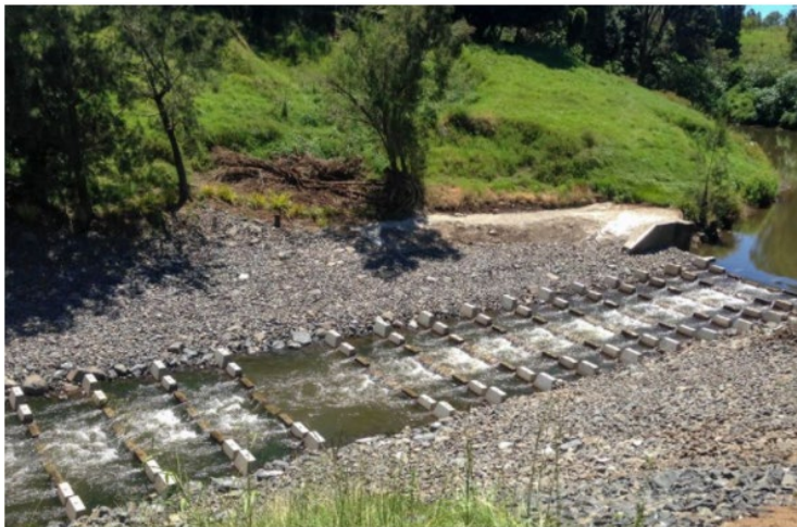
Plate 7: V-shaped rock ramp fishway at Kyogle Weir on the Richmond River
