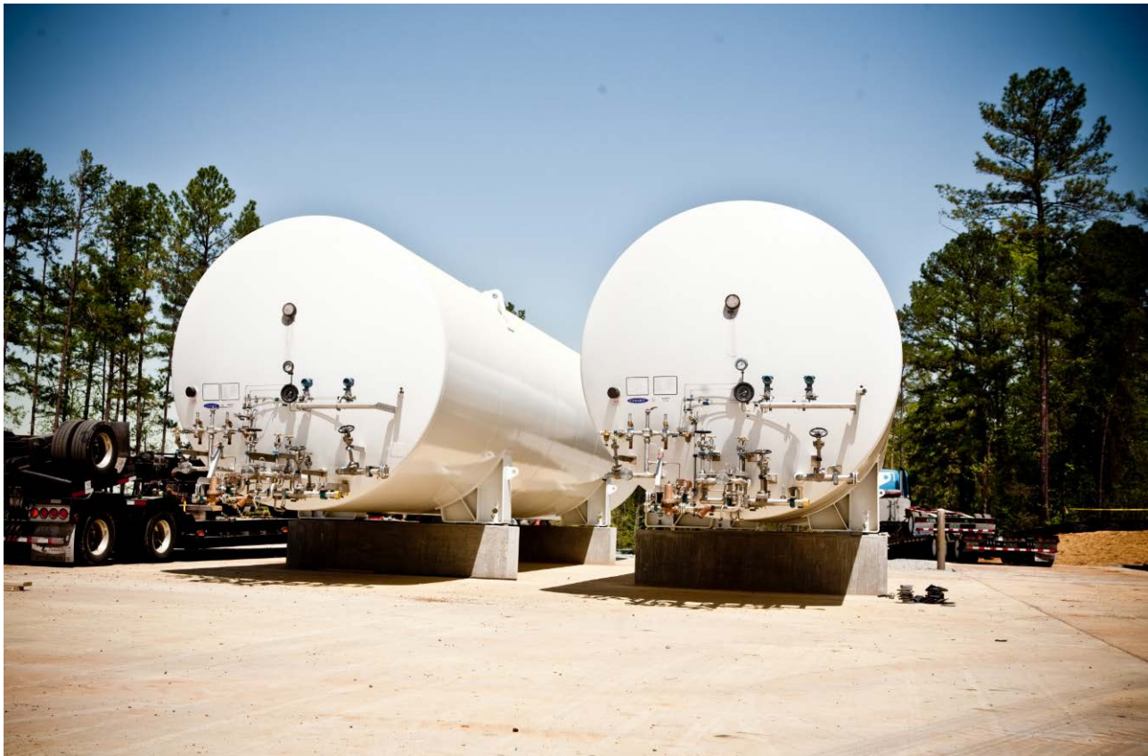
Plate 5: Two 20,000 gallon liquid oxygen tanks installed at Russell Dam, South Carolina as part of large-scale oxygen injection project
