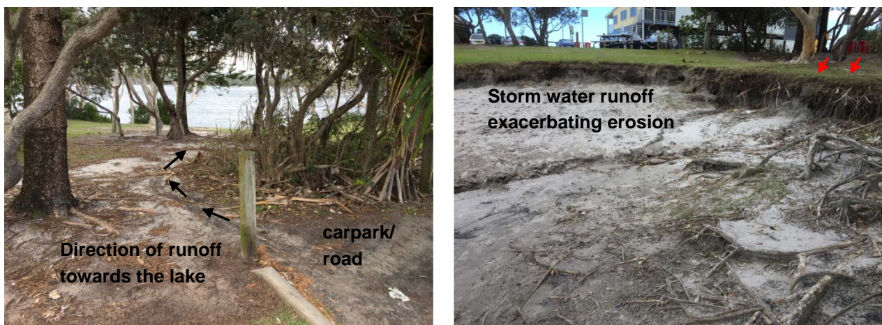
Plate 4: Left - Carpark areas in south-east corner opposite Lennox SLSC showing areas of scour due to stormwater runoff from hard surfaces; Right - Erosion Site 7, downslope of the carpark.
