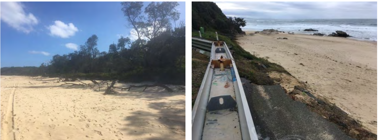
Plate 13: Left: Vegetation debris on receding shoreline north of Swimming Creek entrance (December 2018); Right: recession of beach at Ulrick Drive carpark (north end of Beilby’s Beach) causing undercutting and collapse of the road surface (July 2018)
